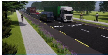
Provision of Segregated Active Travel measures parallel to the existing N24 improving safety for vulnerable road users.
